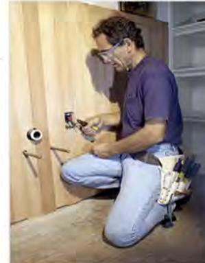
Electricians often cap wires before installing an outlet.
